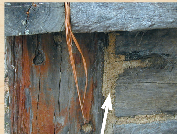
Subterranean termite “mudding” – termites pack mud into gaps in the timber.
