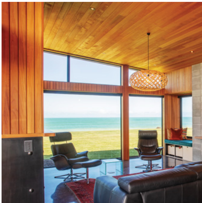
Above right and below: Sequoia sempervirens interior panelling and sarking in a Hawke's Bay house.
