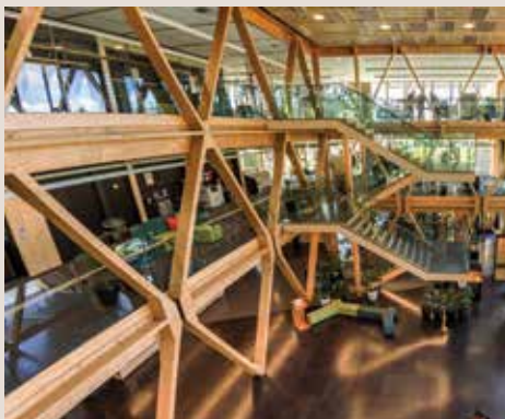
The three-storey Scion building in Rotorua – Te Whare Nui o Tuteata – features a world-first engineered timber diagonal grid structure.
