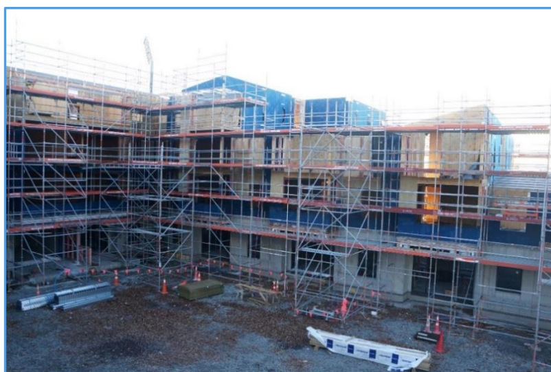
Figure 1: Multi storey rest home in Cross Laminated Timber
